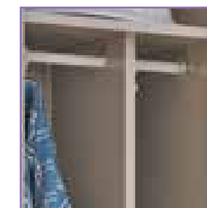
internal partition wall (in 400 mm wide modules)
